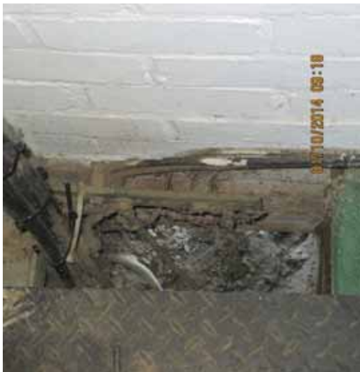
(a) An opening viewed from inside (Stone)
